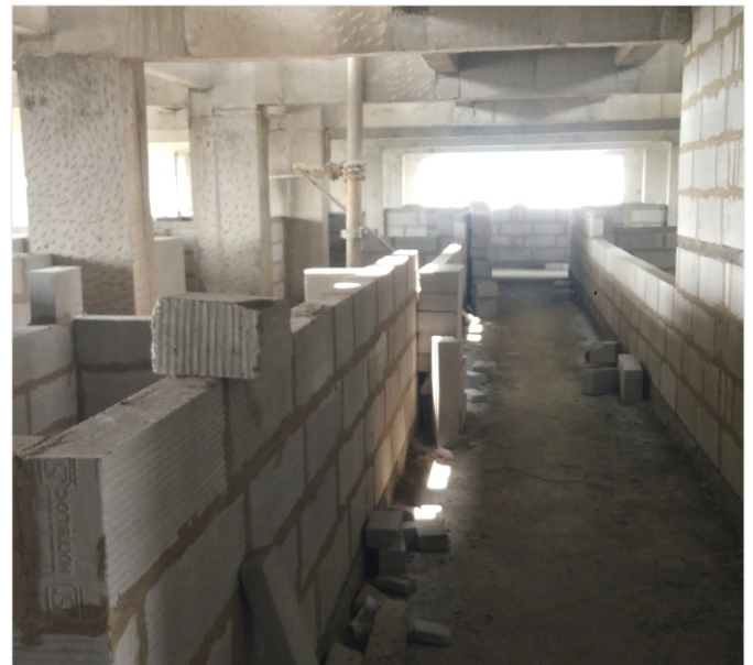
Blockwork is in progress on the 8th floor.
