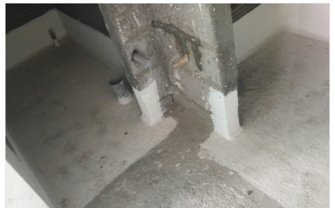
Waterproofing on the 5th floor is in progress.
