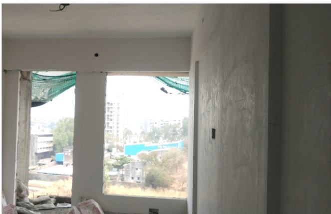
Gypsum work on the 7th floor is in progress.
