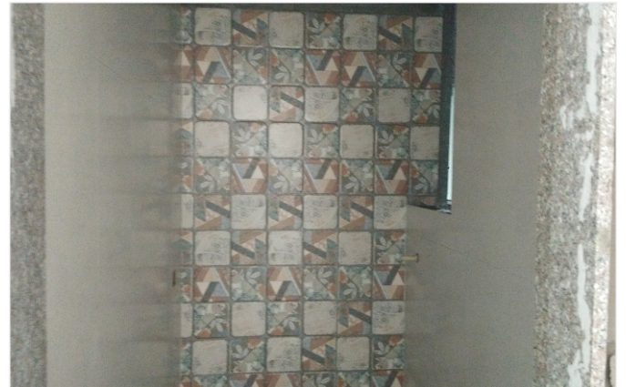
Toilet dado work on the 2nd floor is in progress.
