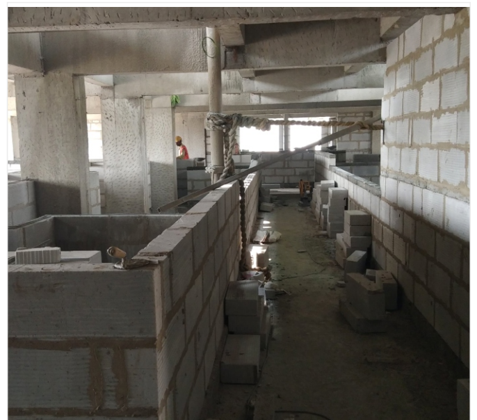
Blockwork is in progress on the 3rd floor.
