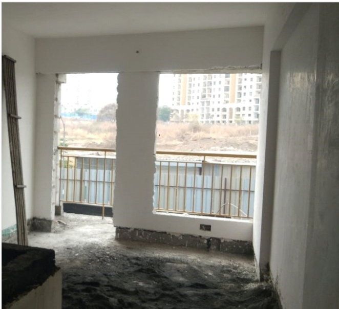
Gypsum plaster, internal plaster, and waterproofing works are ongoing on the 1st floor.
