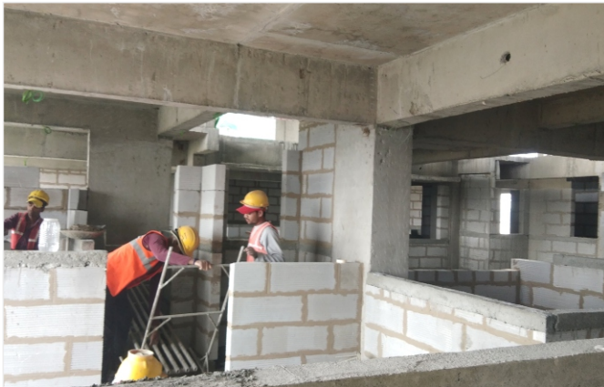
Blockwork on the 8th floor is in progress.
