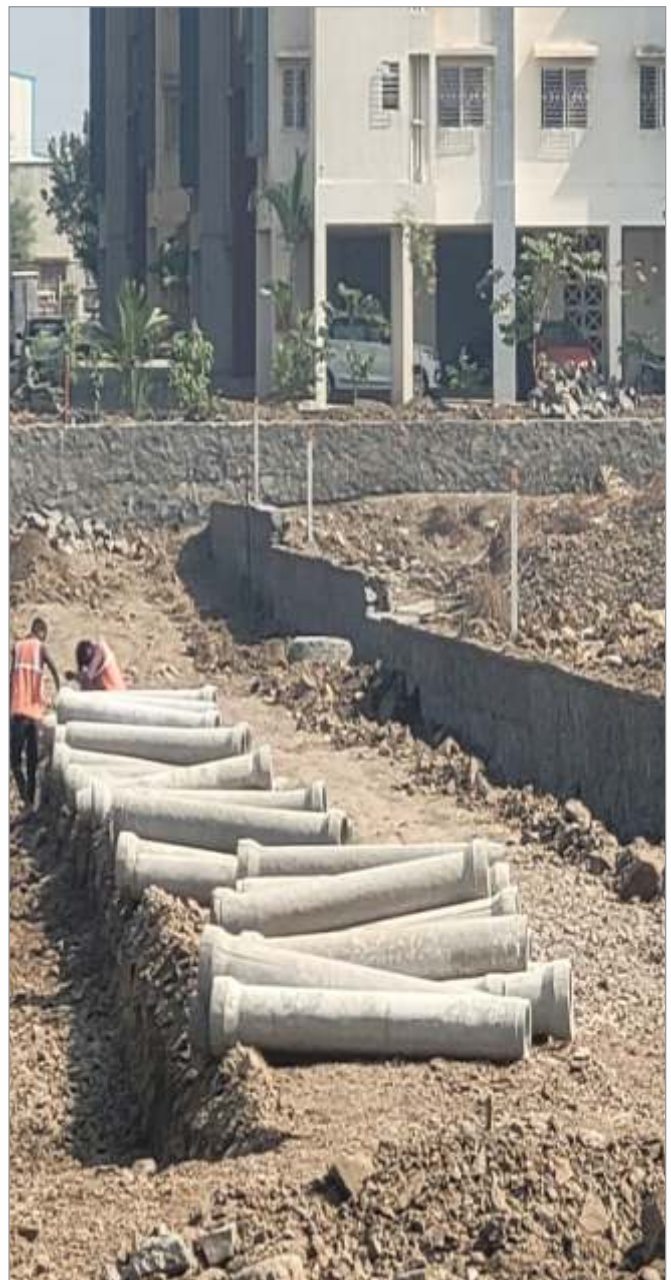
AVASA GROOVELAND - SERVICES WORK
