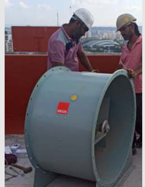
Lift Cladding & Pressurization fan installation work
