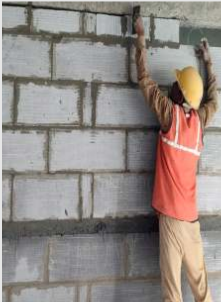
Avon B3 – 20th Floor Blockwork In Progress
