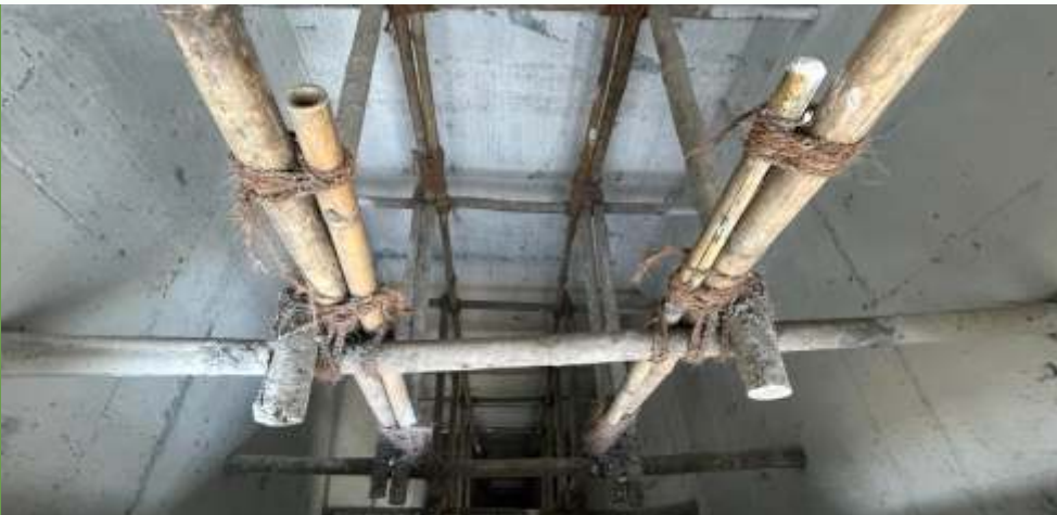
13 Passengers lift shaft white wash done, Electrical work started
