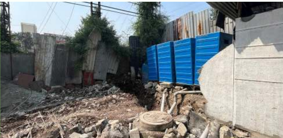
VIP road side balance compound wall excavation done.
