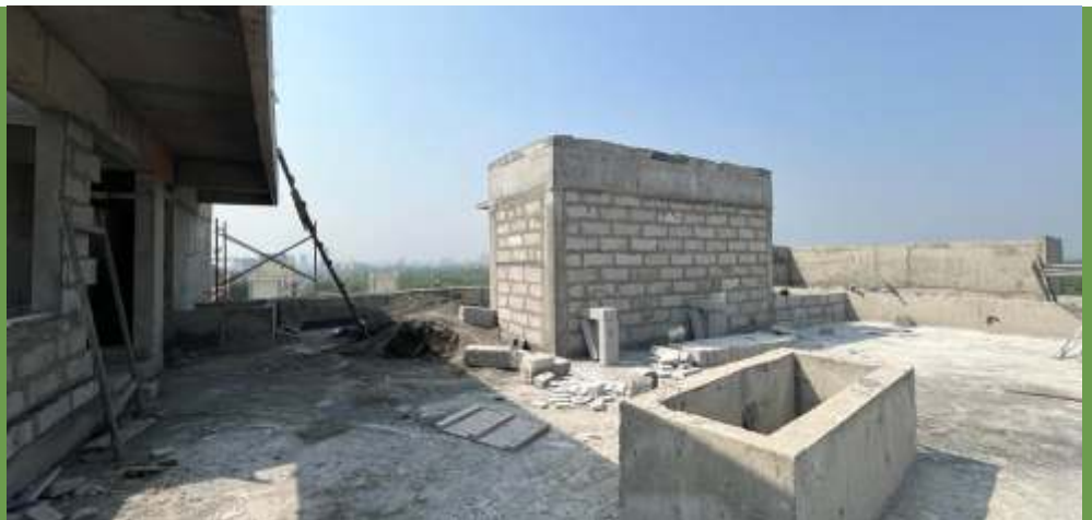
701 Private terrace staircase cap block work done
