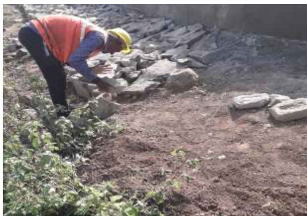
Kutumb – Fruit Forest Stone Pitching & Fabrication Work
