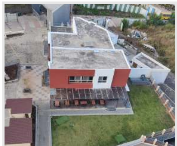
Club House Top View Work In Progress
