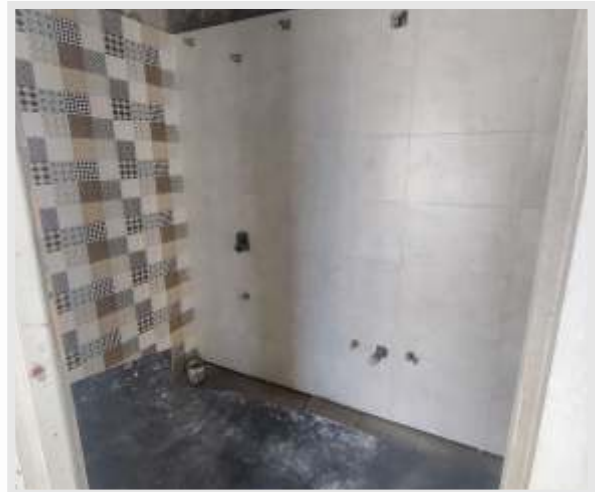
A2 Building 3 rd Floor Toilet Dado Work In Progress
