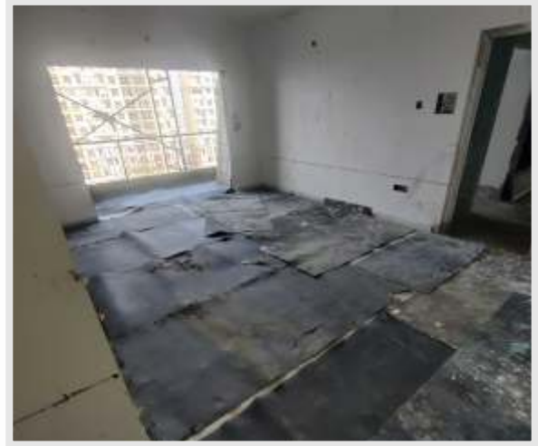
A2 Building – 5 th Floor Flooring Work In Progress
