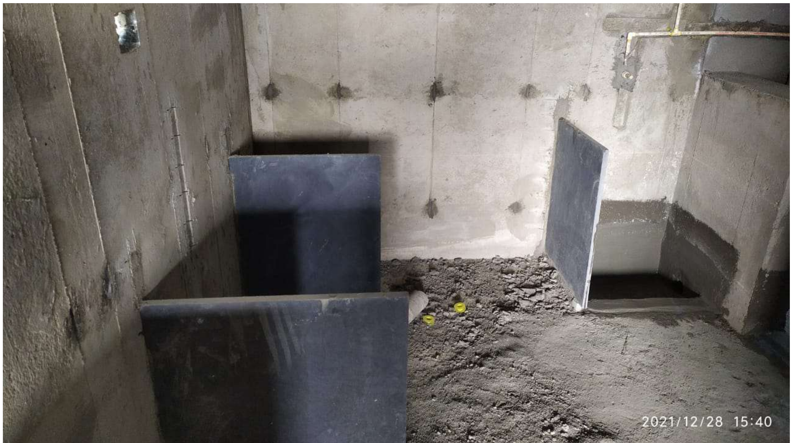
TOWER - A, 9 th FLOOR KITCHEN KADDPA VERTICAL FIXING COMPLETED
