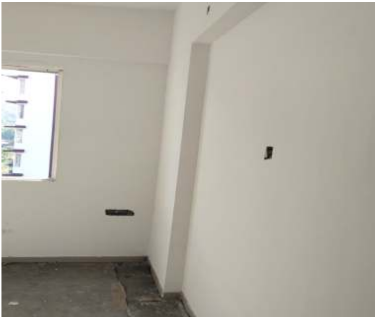
Neelaya C- 10 th Floor Putty Work
