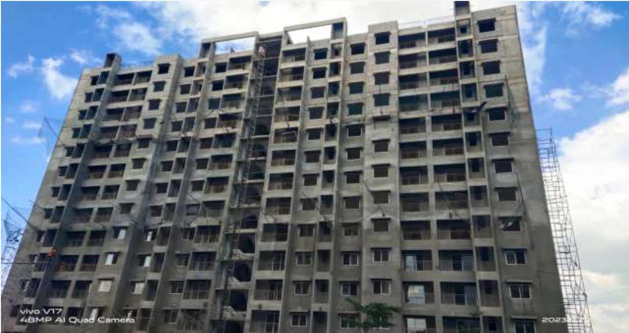
Top terrace plaster work in progress
