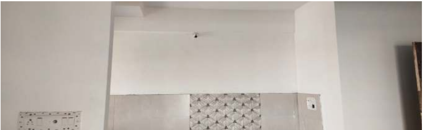
Neelaya C- 5 th Floor First Coat Painting Work
