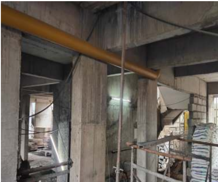
Neelaya C- Fire Fighting Riser Work
