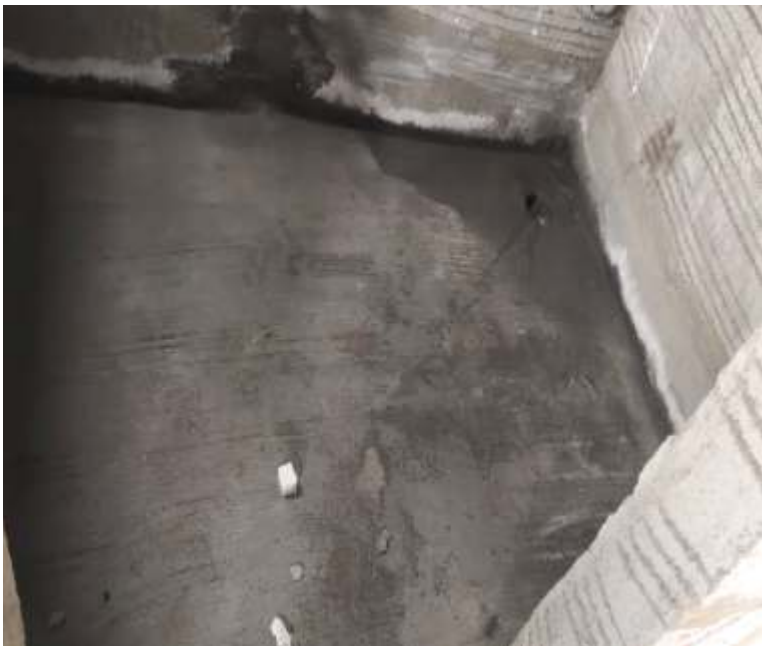
Neelaya C- 14 th Floor Waterproofing
