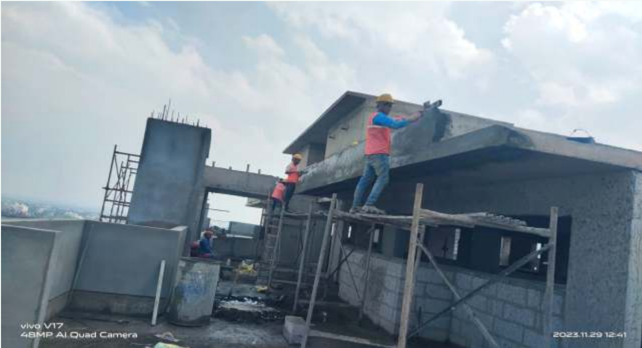
Top terrace plaster work in progress
