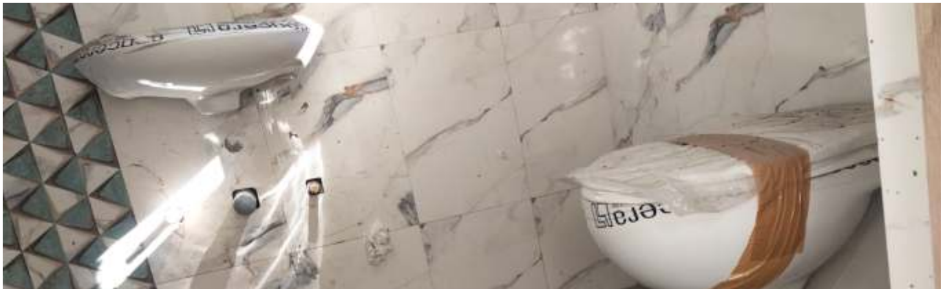
Neelaya C- 7 th Sanitary Fixing Work
