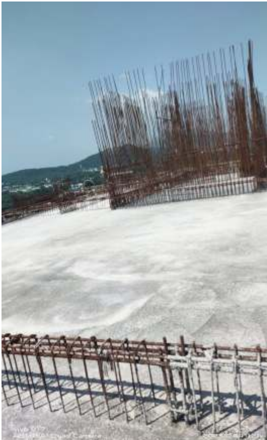
'C' Building OHWT bottom slab casting completed
